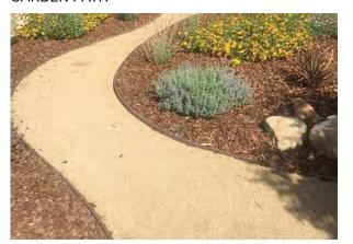
DECOMPOSED GRAVEL WITH STEEL EDGE
